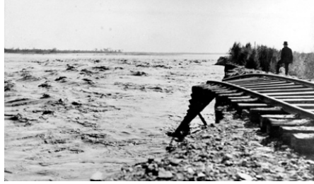
Fig. 6: Colorado River rerouting after the break
