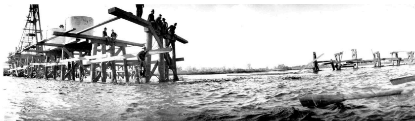
Fig. 7: Trestle construction and rail cars dumping sand to restore the Colorado River
